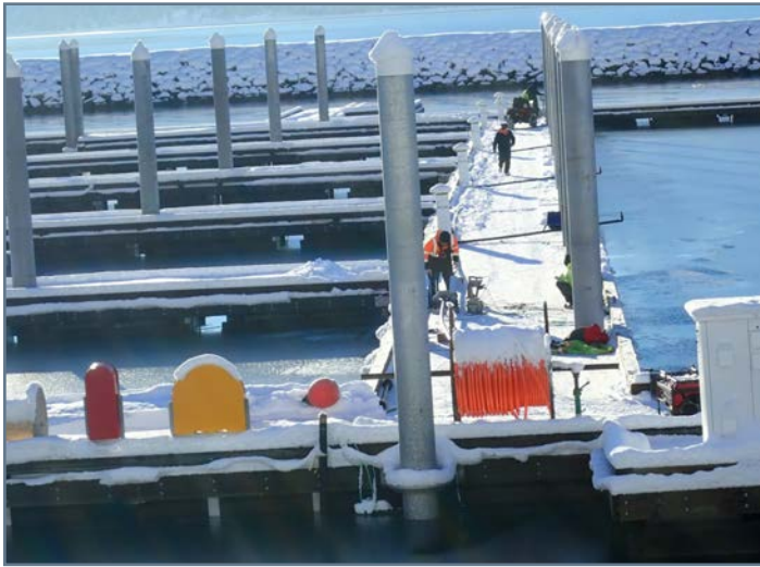
Installing water pipe and power pedestals
