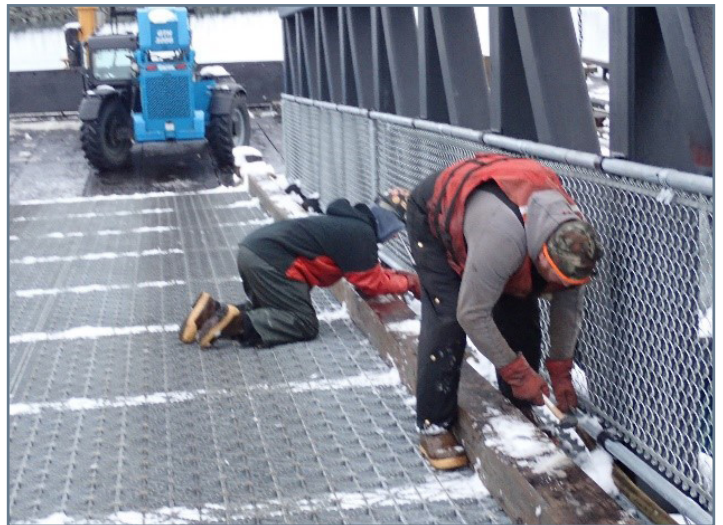
Installing bottom tension rods for fence on DD bridge
