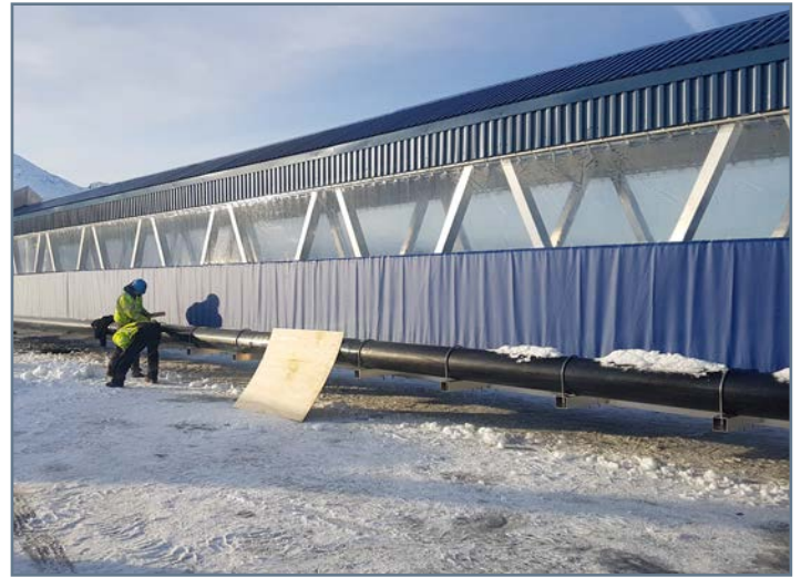
Harris Sand & Gravel installing Arctic pipe on Gangway 3
