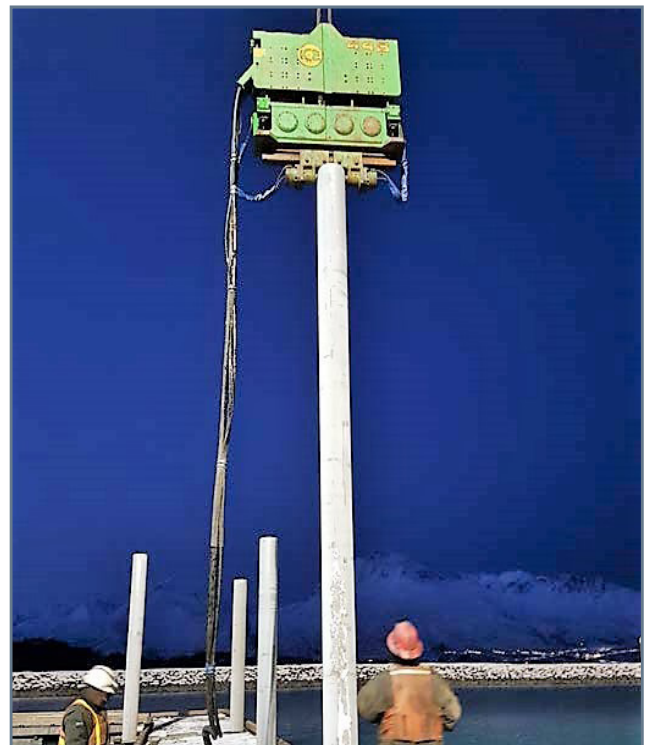
Driving R-Main float pile RM4 with vibratory hammer
