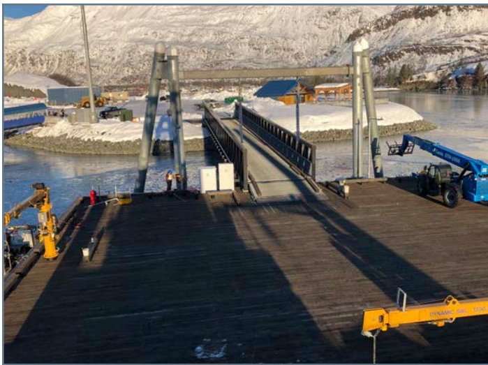
Drive Down Float decking and bull rails are installed
