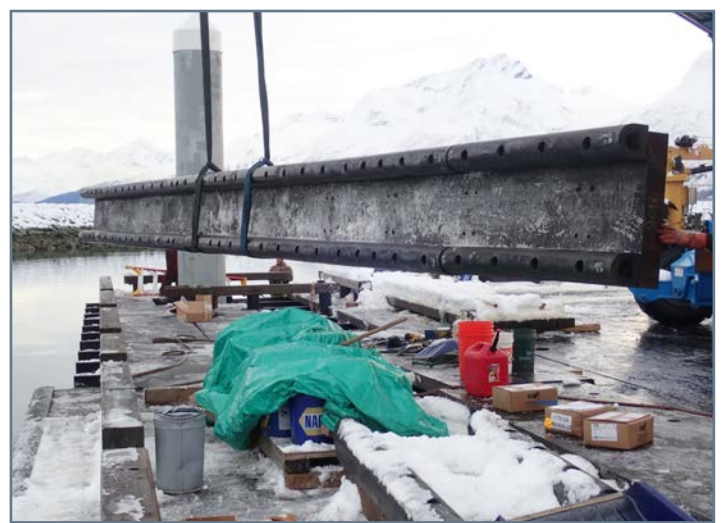
Installing fender assemblies on DD float
