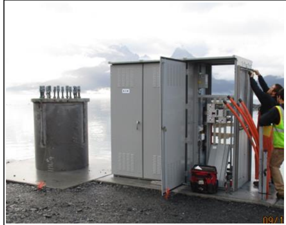
Installing electrical cabinets near east ramp (#3)
