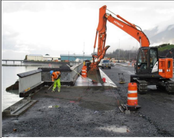
Finish subgrade work at Ramp 2
