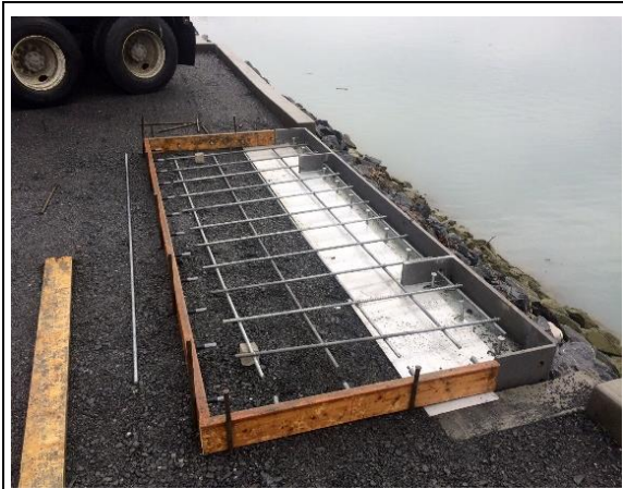
Form and rebar for slab at abutment for Ramp #3
