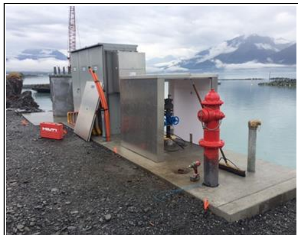
Assembling insulated/heated enclosure around BFP
