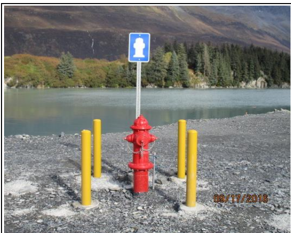
Protective bollards and sign installed at hydrant
