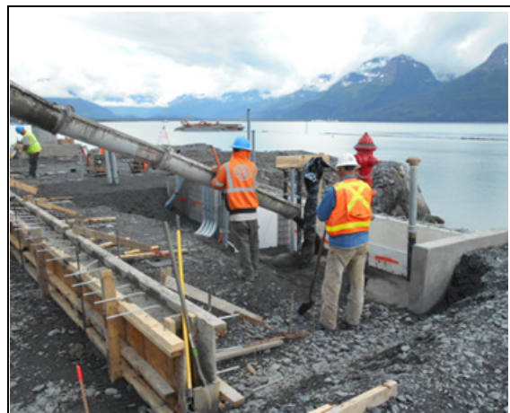
Backfilling BFP foundation with cement slurry
