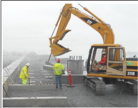
Placing precast concrete sleepers for boardwalk
