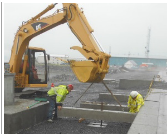
Aligning sleepers on top of concrete pads
