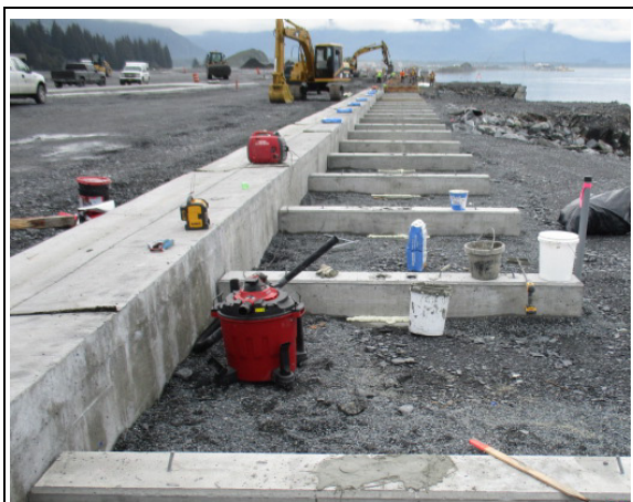
Two rebar and grout secure each sleeper to a pad
