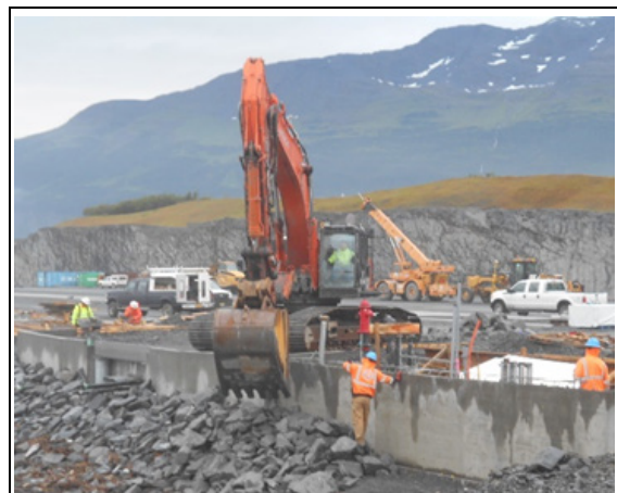
Placing riprap to protect abutment at Ramp #1
