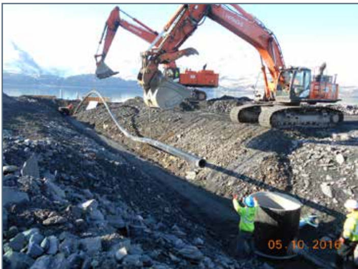
Laying a long section of sewer pipe in trench
