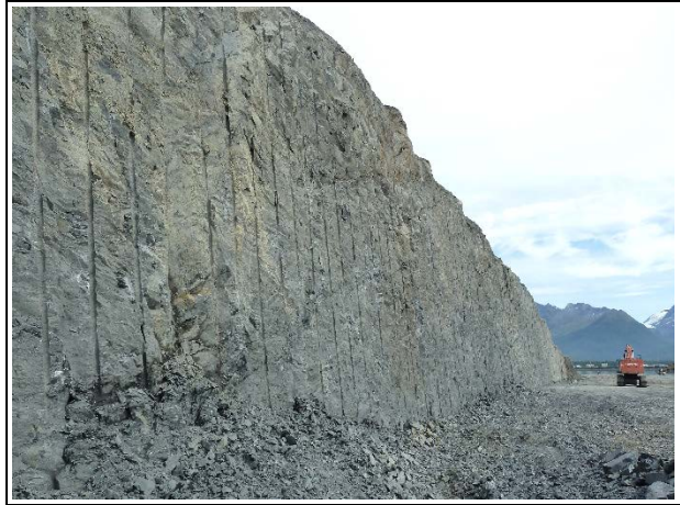
View east along 1:4 face of bedrock after "backsplit" shot
