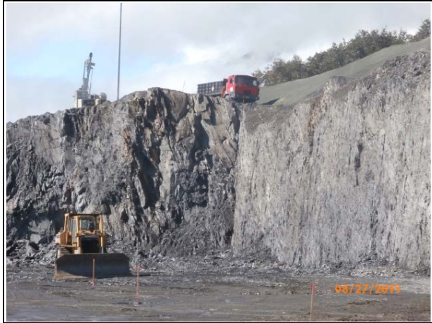
Rig is drilling holes for shot to create 1:4 final slope
