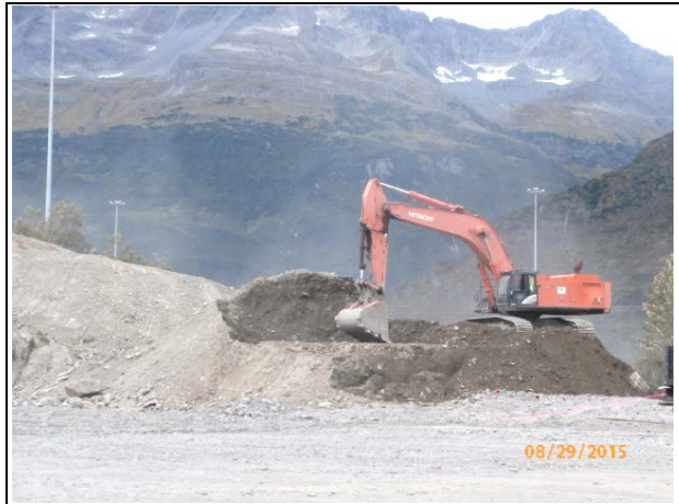
Excavating last of overburden on hill near east access
