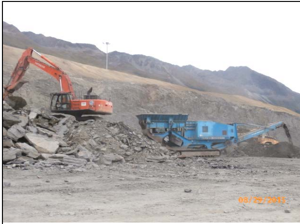
Feeding shot rock into crusher for fill material at east end
