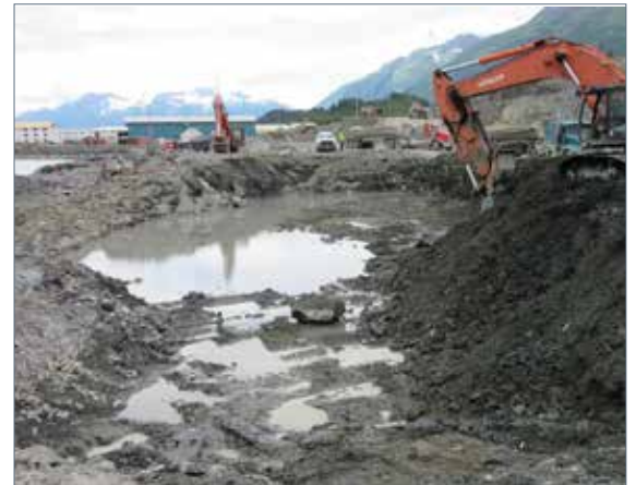
Excavating saturated material below subgrade at bog.
