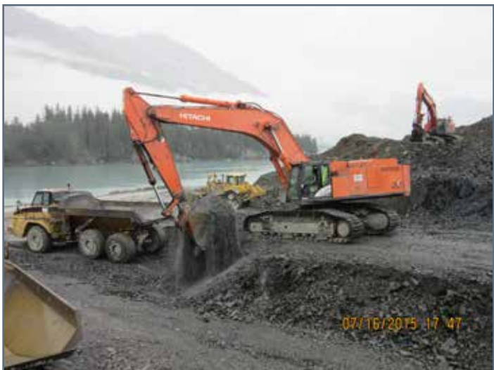
Loading shot rock from east end for fill on the site.
