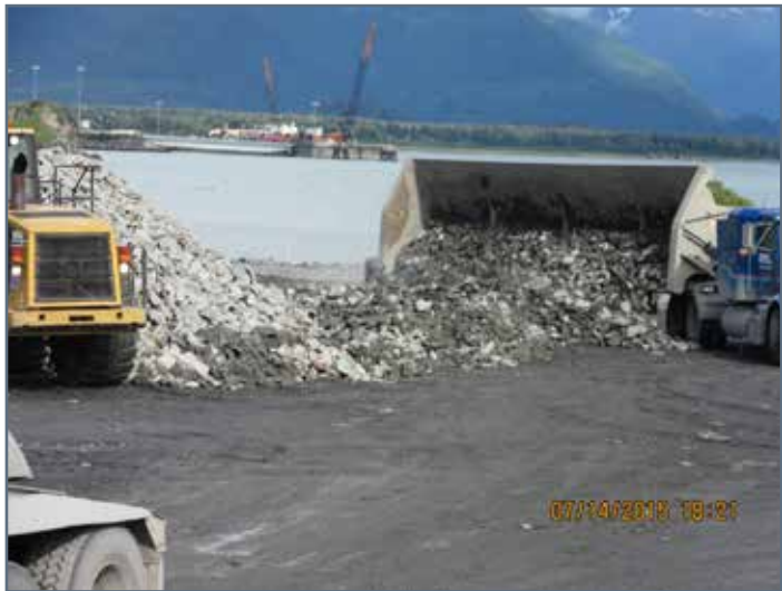
Delivering filter rock from Quarry to stockpile site near tidelands fill.
