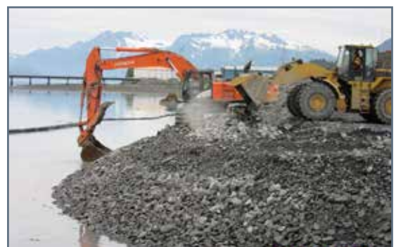
Placing filter rock on slope at SE corner of tidelands fill.
