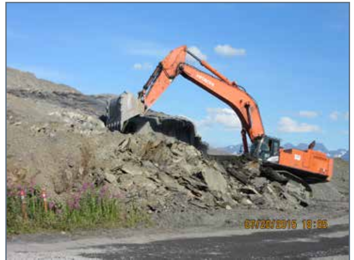
Excavating recently shot rock to widen west entrance.
