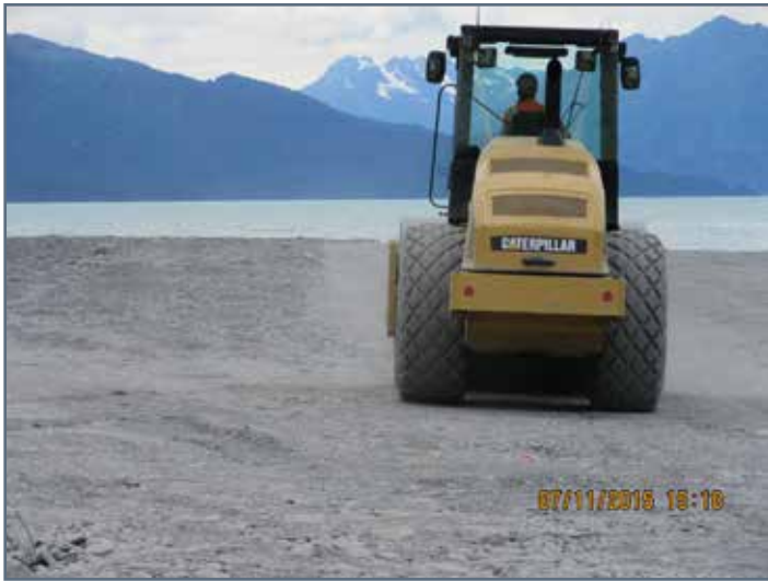
Compacting gravel cover on fill at Sea Otter.
