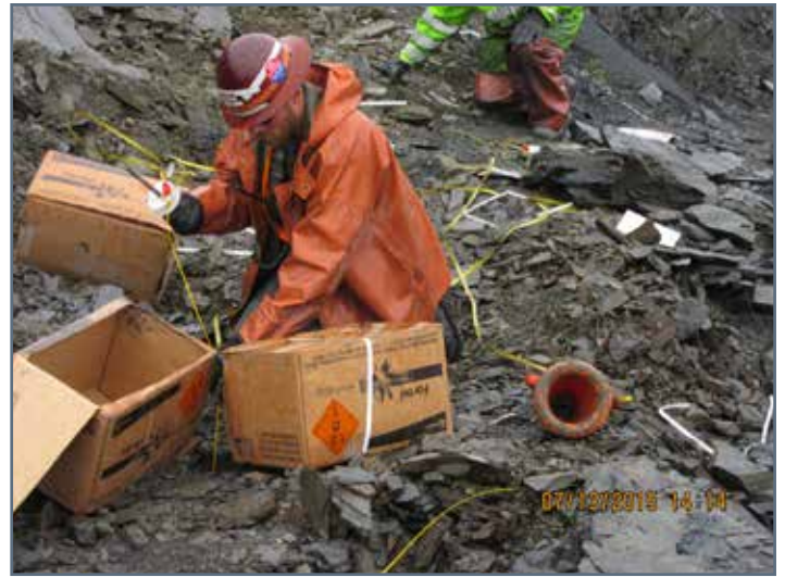
Advanced Blasting placing explosives and detonating materials.
