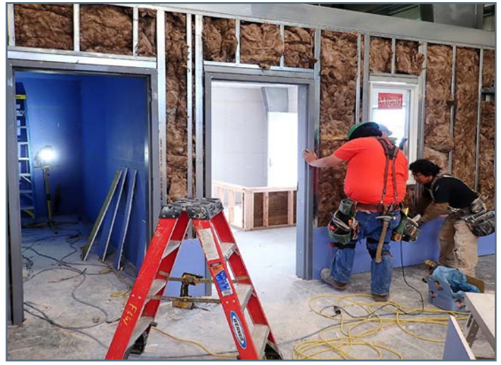
Installing door and window frames in the Warehouse building
