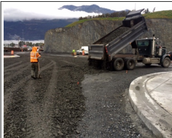
Delivering Type II-A gravel for final subgrade
