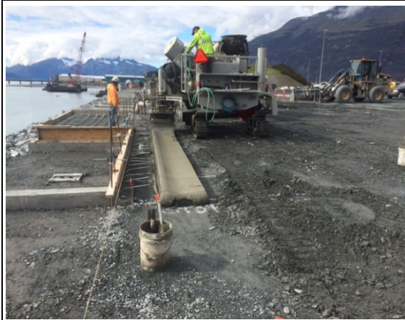
Machine placing curb & gutter at maintenance pad
