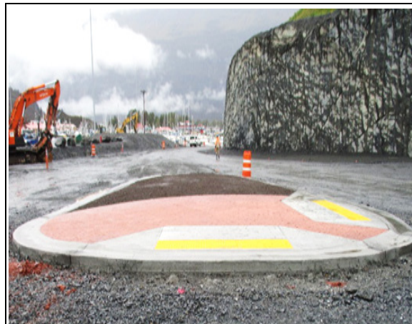
Island separates West Access from launch ramp
