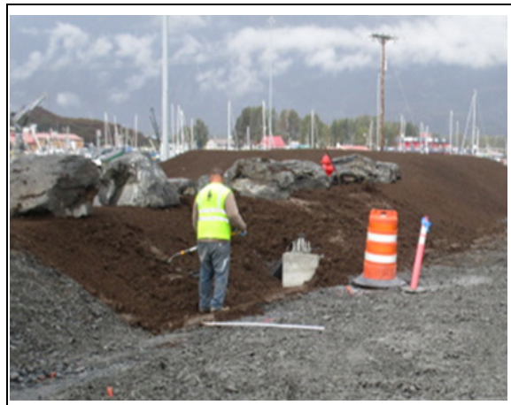
Spreading topsoil on berm along West Access
