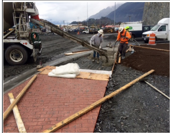
Placing standard sidewalk next to brick imprint
