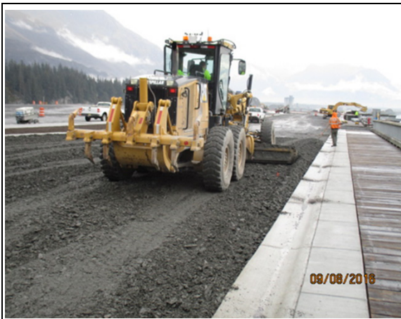
Grading Type II-A to proper elevation along curb
