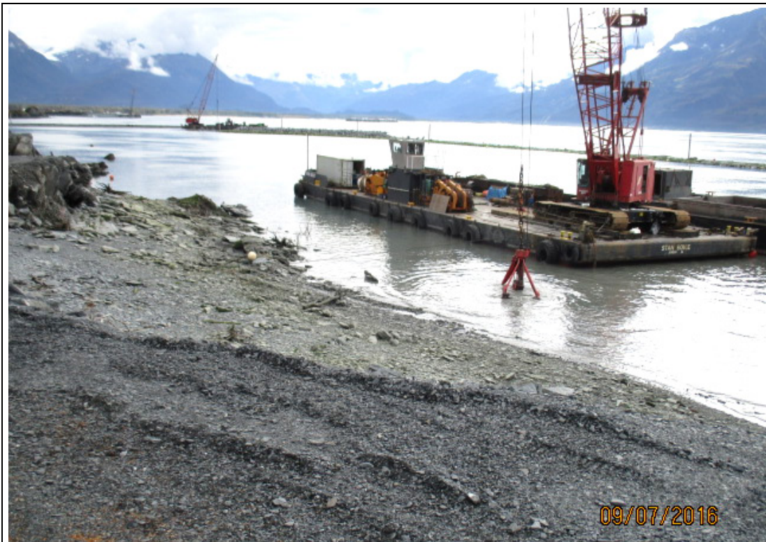
Western Marine dredging sediment along future head float location in northwest harbor basin
