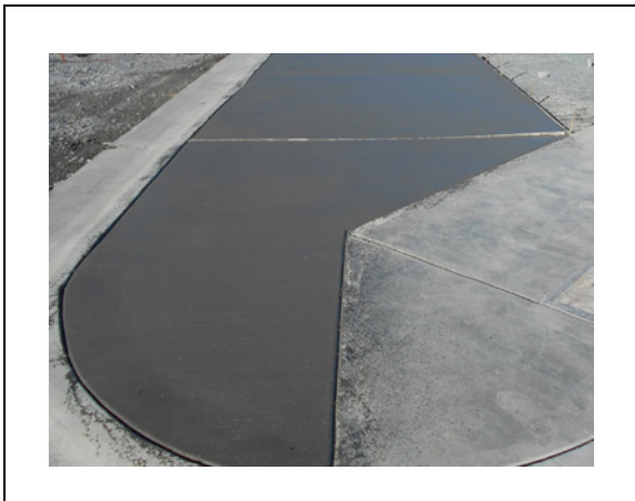
Freshly finished concrete for sidewalk
