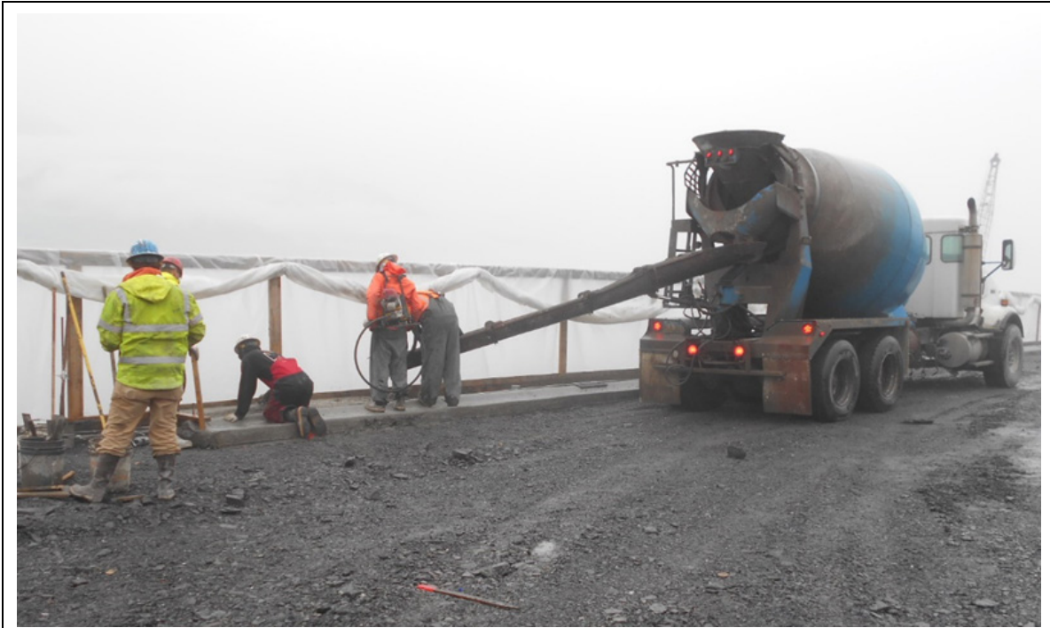
Placing concrete for separation sidewalk between curb and boardwalk
