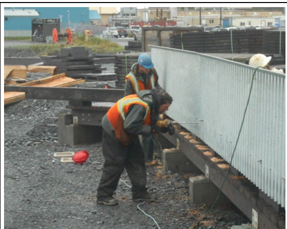
Drilling holes to bolt guardrail to bullrail
