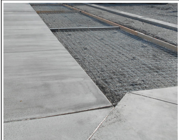
Edge form, control joint and mesh for sidewalk
