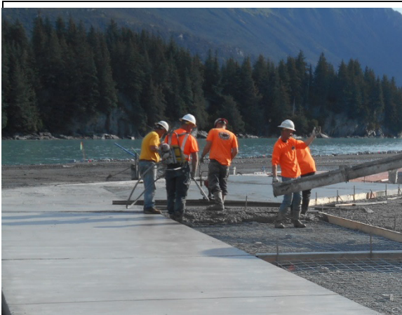
Placing and leveling concrete for sidewalk
