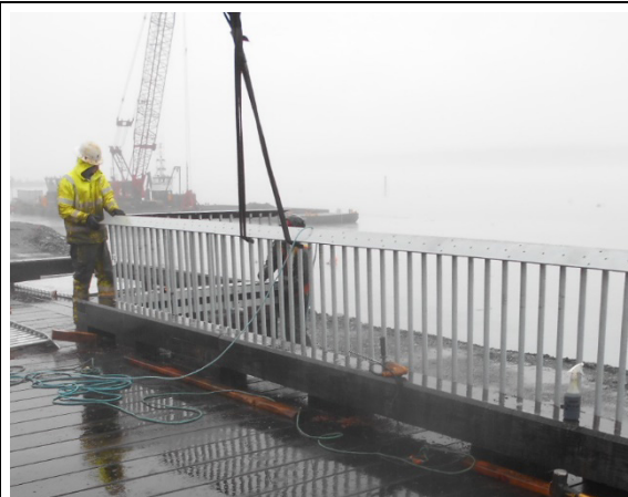
Placing section of guardrail along bullrail
