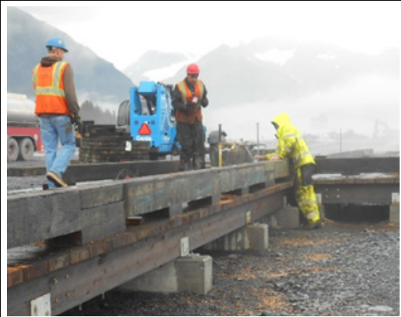
Installing bullrail on top of boardwalk deck
